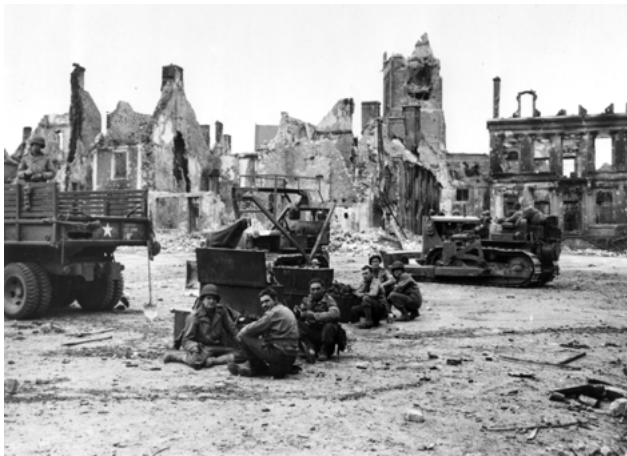
Americans at work preparing Cherbourg for operations. These men are likely U.S. Navy Sea Bee personnel, who specialized in heavy machinery operation and construction work. U.S. Navy photo.
