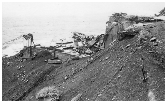
The demise of Scotch Cap Lighthouse. USCG Photo
