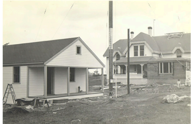
Loran Monitoring building in foreground
